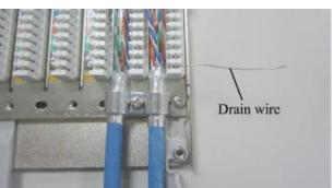
Insert the drain wire into the ninth slot (the slot with no color code) on the IDC connecting block as shown.
