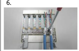
Insert the cable and attach the clip as shown.
